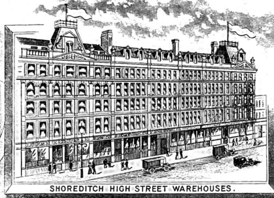
SHOREDITCH HIGH STREET WAREHOUSES.
